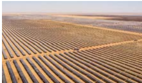
Benban 130 MW Solar Egypt
