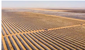
Benban 130 MW Solar Egypt
