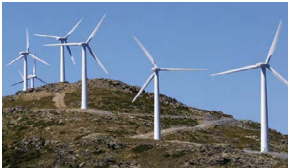
Koudia 100 MW Wind (repowering) Morocco
