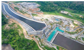
Nachtigal 420 MW Hydro Dam Cameroon
